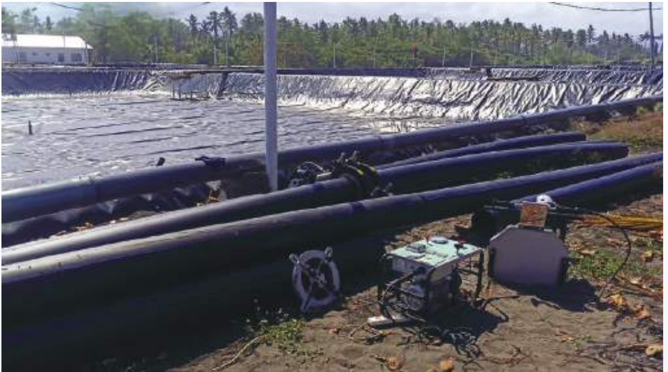
Instalasi pipa HDPE
